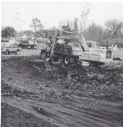
Pond excavation — from plans to the field.
