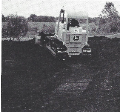
Sometimes outside contractors and equipment are needed for construction.
